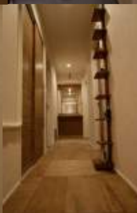
APARTMENT Interior Renovation
